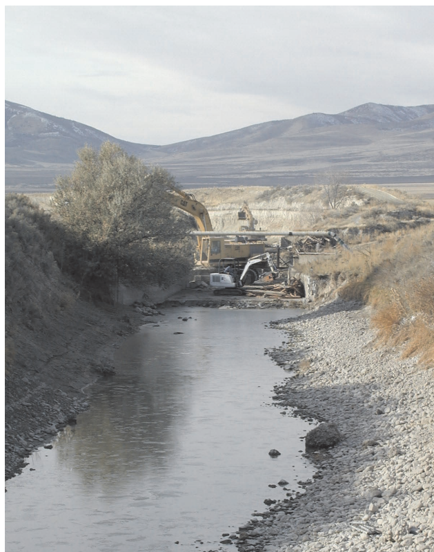
Canal Maintenance in Box Elder County
