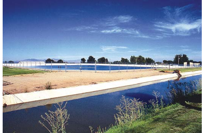
Secondary water reservoirs like this one in Davis County are an important component of the extensive secondary irrigation systems within the Weber River Basin.
