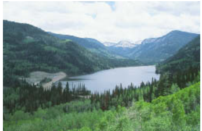
Surface water reservoirs, such as Smith & Morehouse Reservoir shown above, are a familiar element of many water developments.
